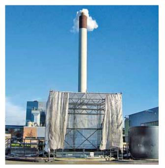
The covered station for dumping the shredder fibres
